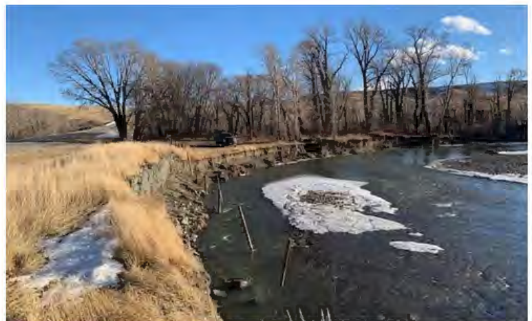
Looking downstream (south) between US-89 and Two Medicine River prior to construction contract award (November 20, 2020). Credit: Paul Sturm
