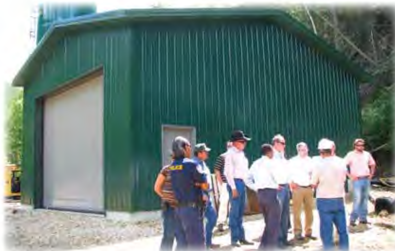
Standing in front of the Water Treatment facility on the Fort Belknap Reservation, Governor Schweitzer and Fort Belknap President Tracy King are briefed by Department of Environmental Quality staff about the water treatment process occurring at this Swift Gulch drainage site
