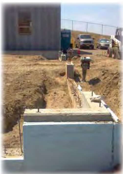
Foundation walls being poured at the Montana Department of Transportation storage site in Busby on the Northern Cheyenne Reservation (Photo by Cody Mitchell)
