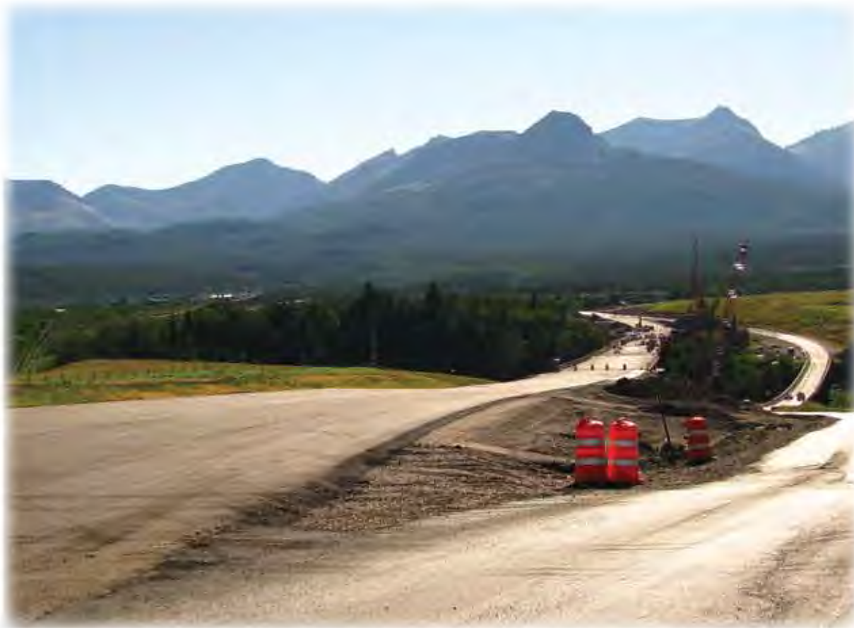
The new Two Medicine Bridge located on the Blackfoot Reservation nears completion – many tribal members were employed during the construction period
