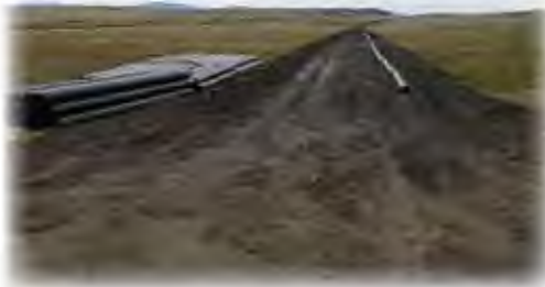
Blackfeet Water Project Phase III—laying connecting pipe (Photo by Lesa Evers)
