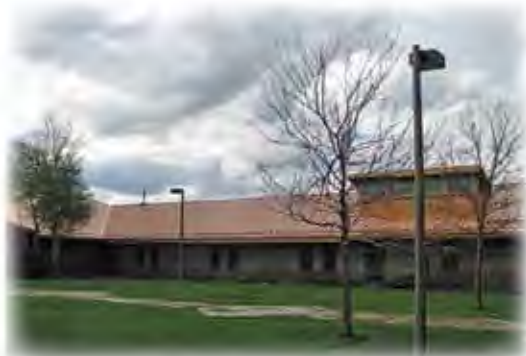
Northern Cheyenne Tribal Building Roof (Photo by Lesa Evers)
