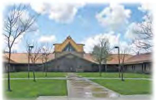
Northern Cheyenne Tribal Administration Building roof improvements
